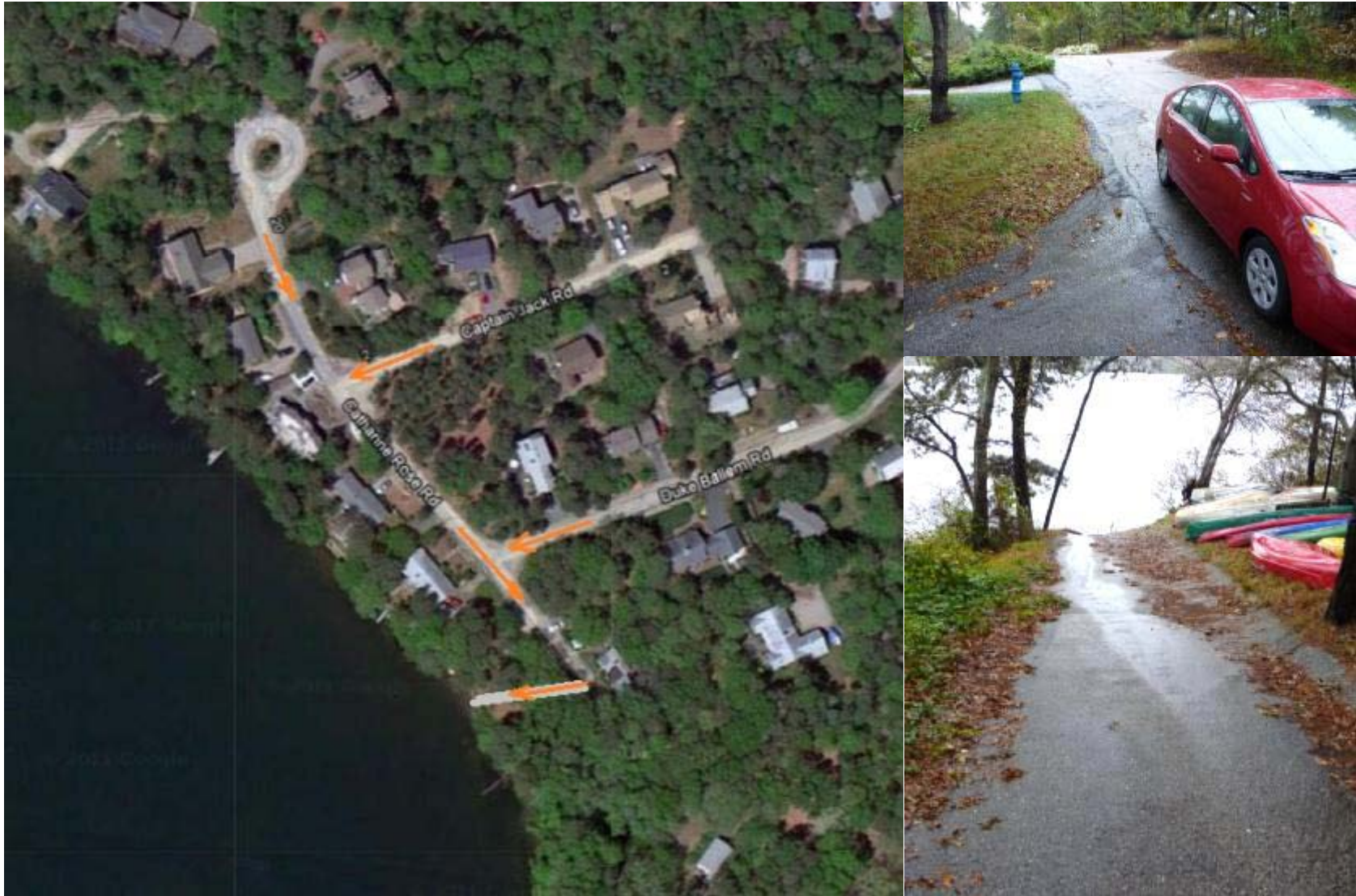
Figure 13. Runoff and erosion hazard at Catherine Rose Road.
